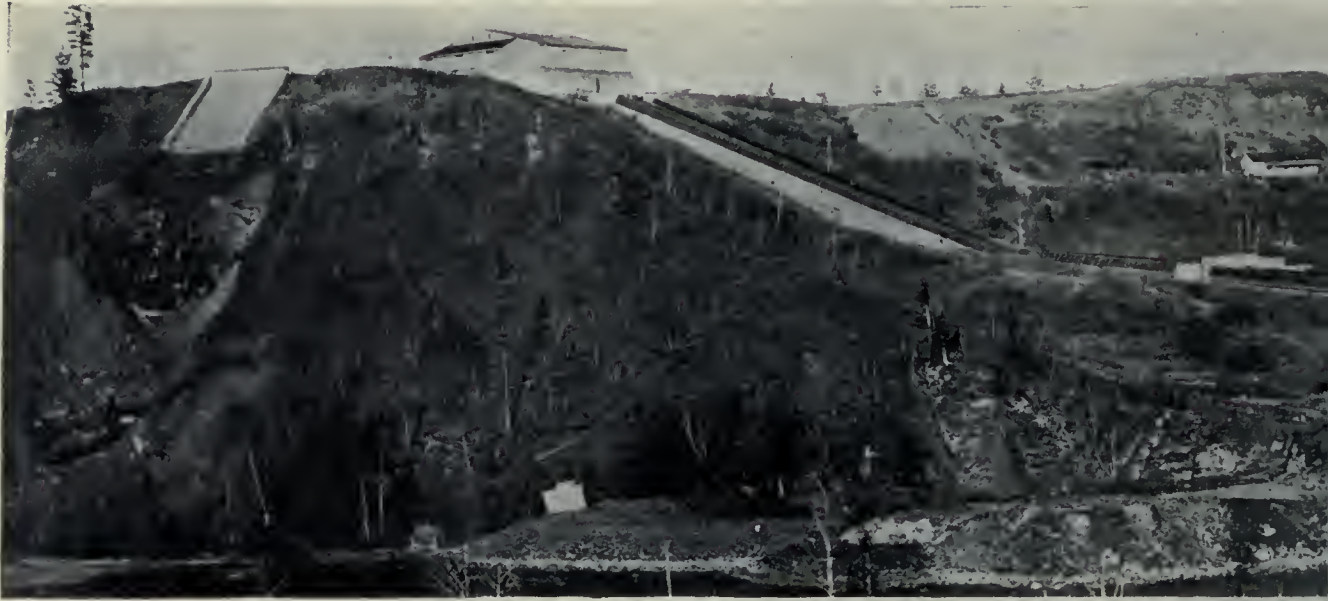
General View of the Kaministiquia Power Company's Hydro-electric Station at Kakabeka Falls—Shows Forebay and Spillway
